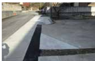
既設水路改修
